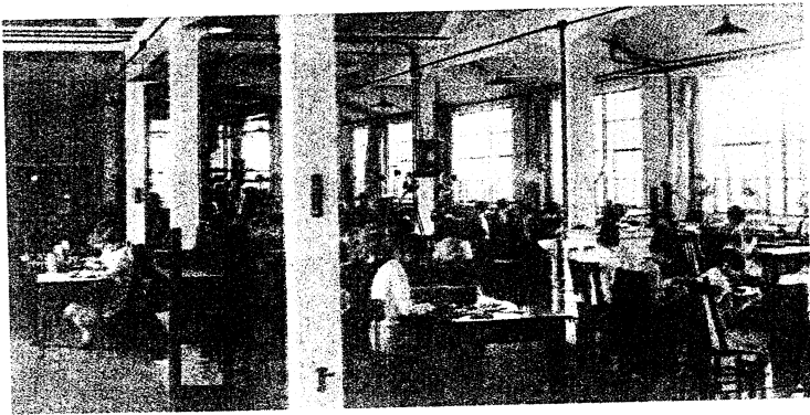
The Assembly Department was one of the first to move into new quarters in the Morrison Plow Works building. Some remodeling was necessary after the building was purchased in 1917 and, during the first years, only a part of the available space was used by the fledgling Sheaffer Pen Company.
